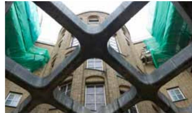
NARROW SEAMS IN THE CONCRETE BETRAY WHERE THE FORMWORK ELEMENTS WERE ATTACHED TO EACH OTHER. THEY WILL BE FINISHED INVISIBLY AT A LATER STAGE.
